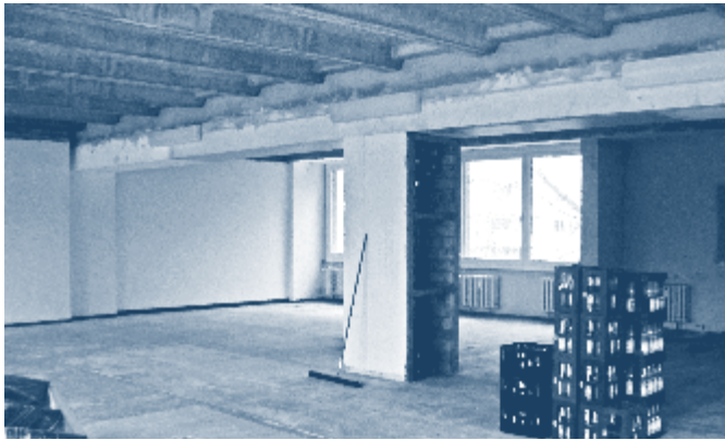
The new salon in the ND building: from a storeroom to a representative space for events
